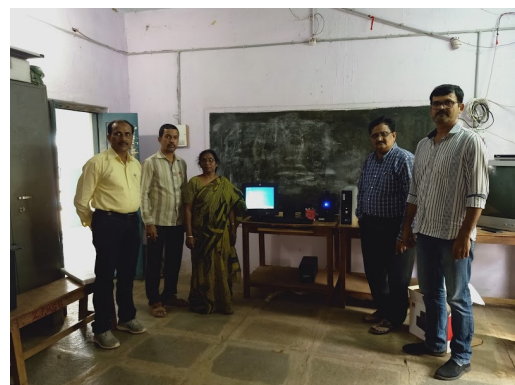
During installation of computers at ZPHS, Budhera
